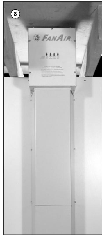
**STEP 9** From the outside, slide in the evacuation pipe and adapt it to the elbow of the fan casing. This will show you where to cut the length of this pipe to finalize the installation of the outside vent.
